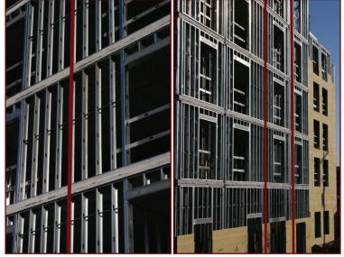
Example of framing aligned vertically. The red lines trace the axial Trusses bearing on the studs, which are aligned vertically to the load vertically from the roof to the foundation.
